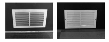
When the flow is limited or inaccessible between rooms downstairs (if there are walls or partitions), then install a grille 10" x 14" (or other grill configuration, having total area of not less than 100 sq. in.) in the bottom of the door or wall to avoid having stagnant air in those areas. Otherwise interior doors must remain open. This insures that all the air drawn into the Humidex comes from all areas of the basement.
